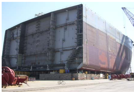
Fore body built on slipway
